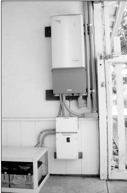
(left) A power center with backup storage batteries is located in a shaded porch area. (right) A combiner box combines DC circuits from several PV panels.
