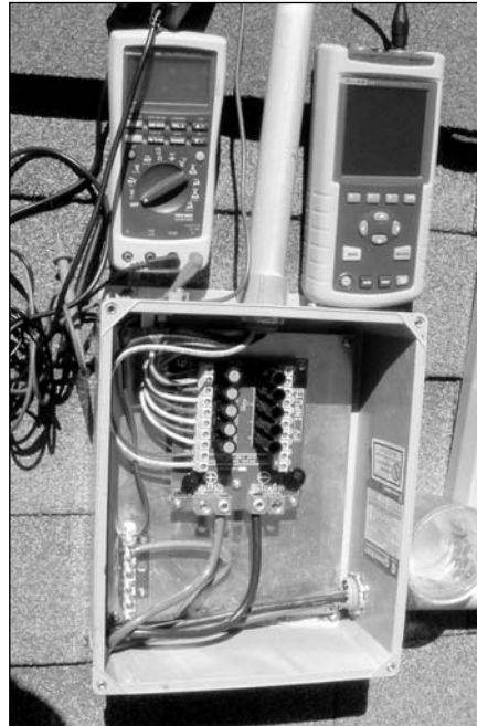
(left) A power center with backup storage batteries is located in a shaded porch area. (right) A combiner box combines DC circuits from several PV panels.
