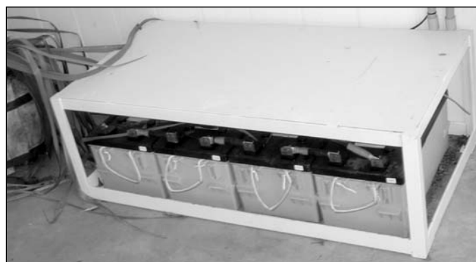
(top) This rooftop mounted PV system has arrays facing south and west. (bottom) These storage batteries provide uninterrupted operation of critical electrical loads even when power from the grid is unavailable.
